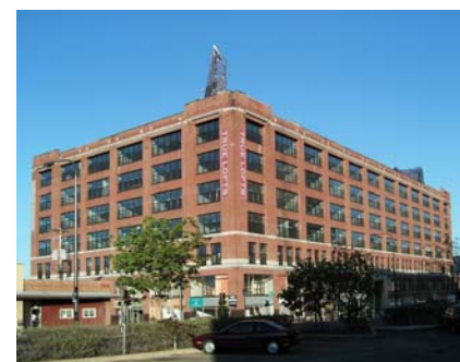
Foot, Schulze & Co. Building after renovation
