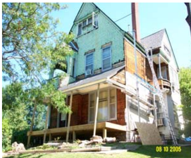
House in Dayton's Bluff District during rehabilitation
